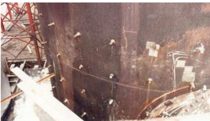
2. Nipples were welded on tower body as well as gas inlet.
