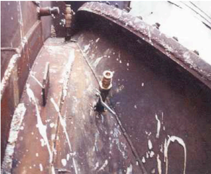
5. T valve gate with quick connect coupling is screwed onto threaded nipple.
