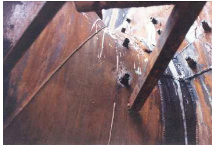
3. Threaded nipples so plugs can be put in after pressure grouting.
